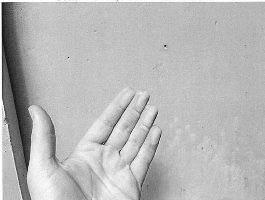
Moderate to heavy chalking depending upon exposure.
