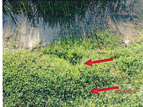
Burrow Causing a Washout
